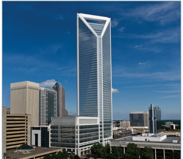
In the Duke Energy Center in Charlotte, N.C., 16 separate building systems, including three building automation systems, are integrated on one network.
