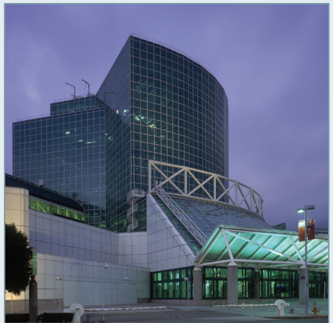
The Los Angeles Convention Center is enhancing its smart building capabilities with upgrades to its ventilation system.
