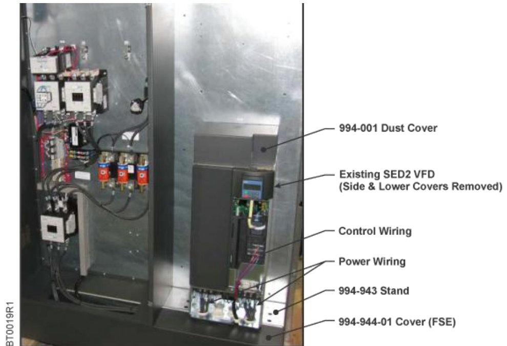
Figure 2. Remove Existing SED2 Drive.
